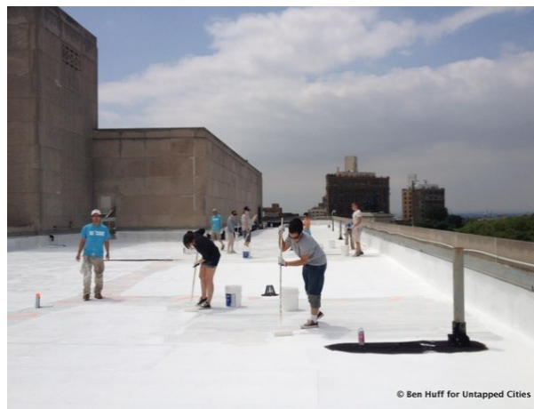
Figure 14 - The white roof project in New York.
