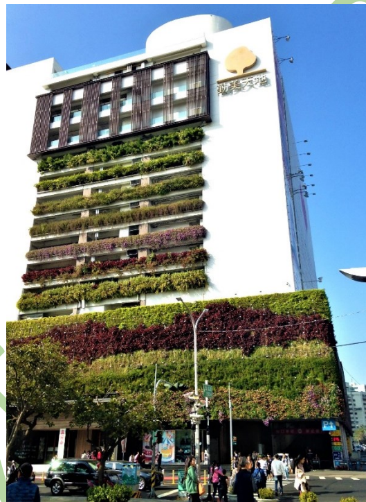
Figure 16 - Park lane by CMP in Taichung, Taiwan
